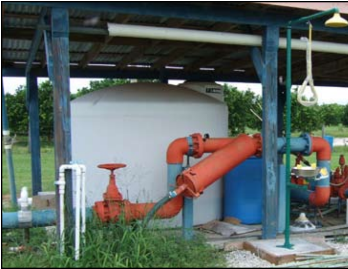
Fig. 6.3. Nutrient solution sources for fertigation are stored in large plastic tanks at the irrigation pump station. (Thomas Obreza)
