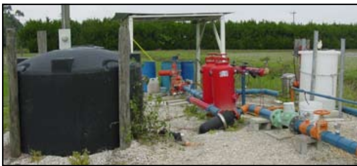
Fig. 7.2. Fertigation equipment, including fertilizer tank (left), filters (center), and injector (right). (Mongi Zekri)
